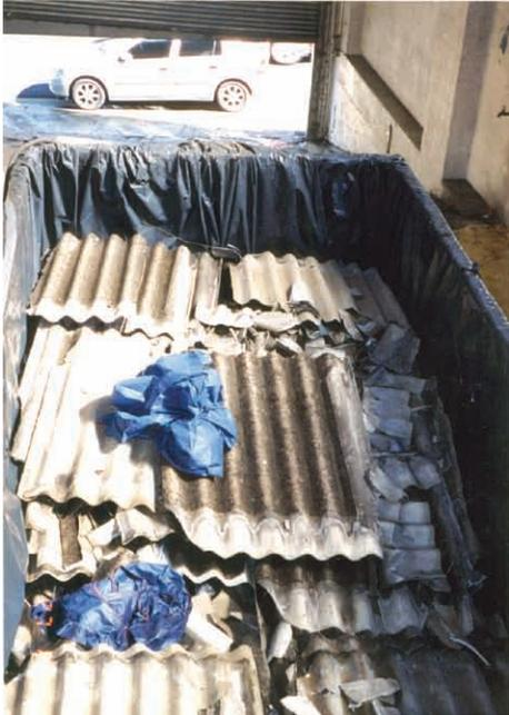
WRAPPED ASBESTOS WASTE
