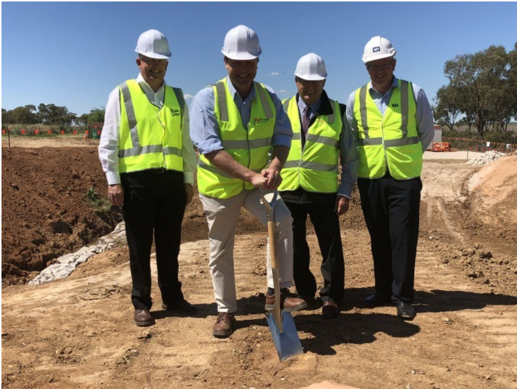
Turning the first sod for the construction of the new automated flood gates at the East Mirrool Regulator at Yenda, (L-R) Griffith City Council General Manager Brett Stonestreet, Austin, Griffith Mayor John Dal Broi and Murrumbidgee Irrigation CEO Brett Jones.
