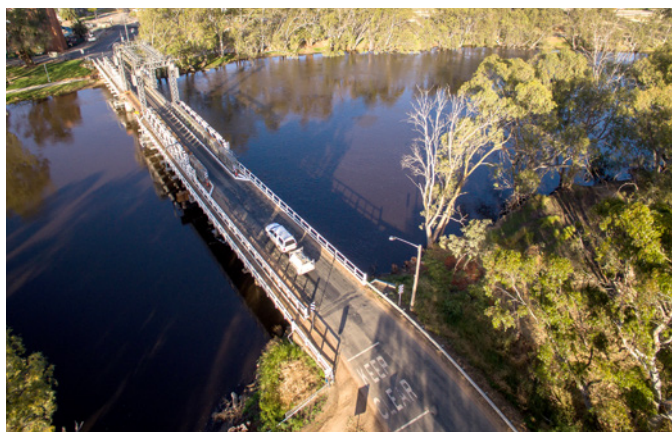
The existing Swan Hill Bridge
