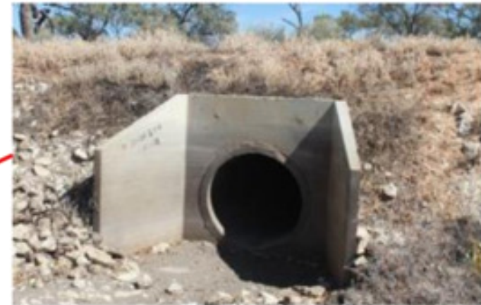
Existing culvert between Waugorah Lake and North Stallion Swamp
