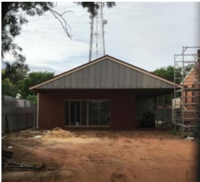
The Creative Learning Centre under construction
