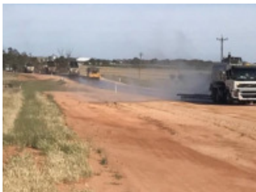
Bitumen sealing, Weimby-Kyalite Road
