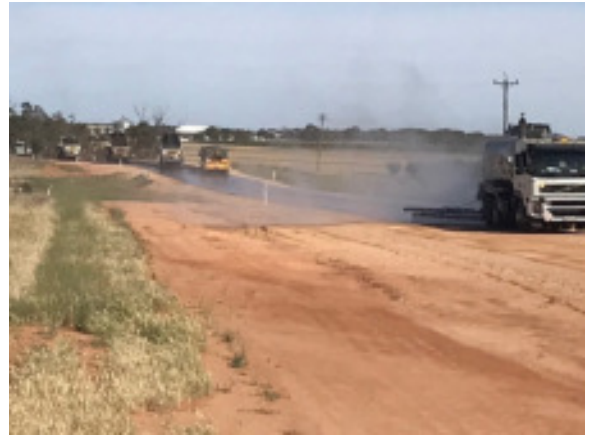
Bitumen Sealing, Weimby-Kyalite Road
