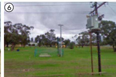
Existing sewerage pump station - Visually intrusive
