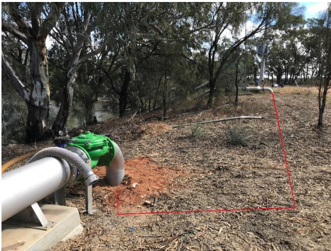
Figure 9 Alignment of connecting manifold
