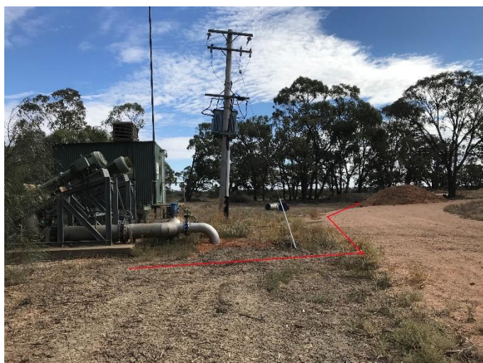
Figure 5 Alignment of delivery pipe
