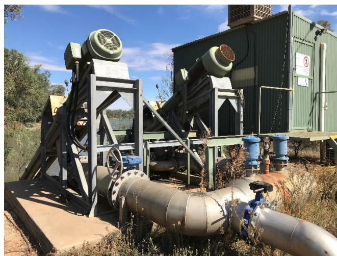
Figure 4 Existing electrical pump station
