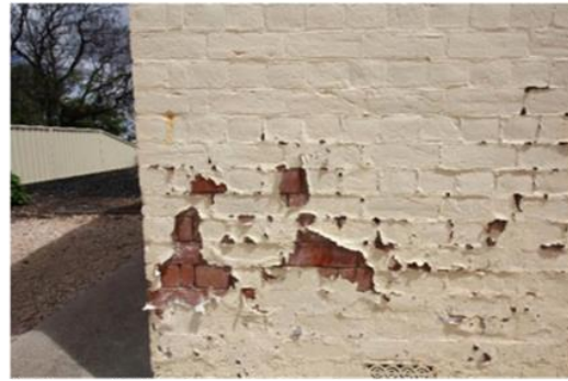
Evidence of rising damp at external wall
