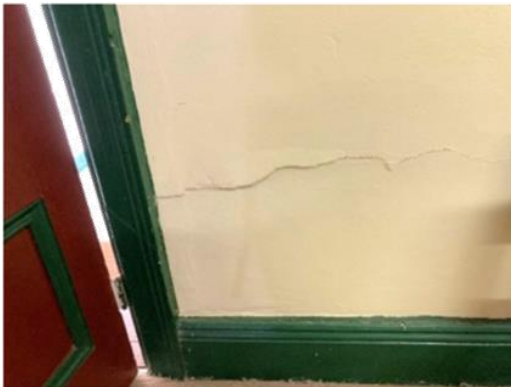
103: Entry Room – cracking at walls
