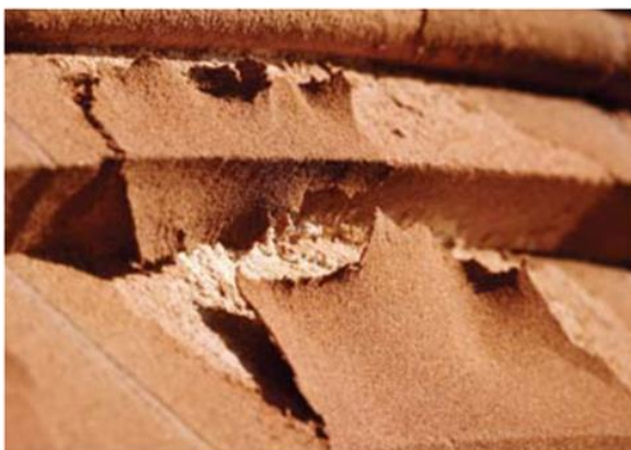
Figure 3 Inappropriate use of water repellent coating, trapping moisture and salts and causing loss of the sandstone's natural case-hardened surface. Beneath this 'skin' the stone can be quite weak.
