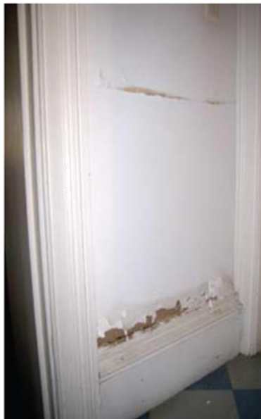
Figure 20 Evidence of previous treatment with hard impermeable plaster. Damp is evaporating from above and below the impermeable zone.
