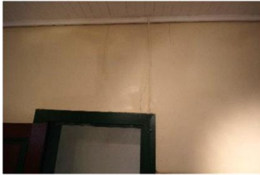
124: Robinvale Room - cracking at walls
