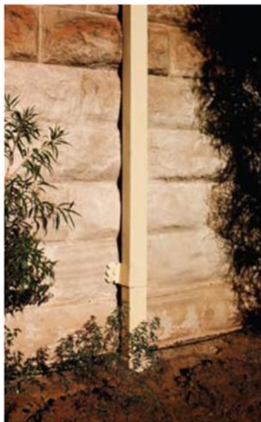
Figure 24 Garden beds against walls almost guarantee salt damp problems. Here the DPC was buried by 300 mm of soil — five courses of sandstone have been severely damaged.
