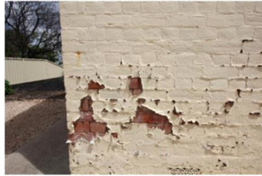
19: South facade showing 'rising damp'
