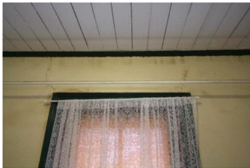
77: Nurses display structural tie rod / cracking
