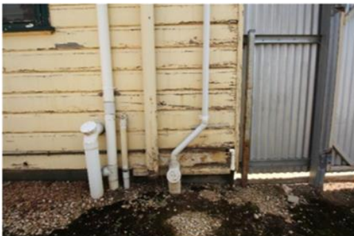
5: View of deteriorated weatherboards
