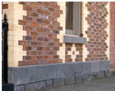
Figure 1 The dense bluestone base courses of this Melbourne building help reduce upward movement of moisture. Dense stones such as bluestones and granites are commonly seen as base courses around Australia.
