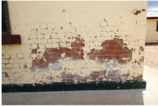
18: South facade showing 'rising damp'
