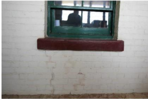
144: Infill verandah cracking at wall
