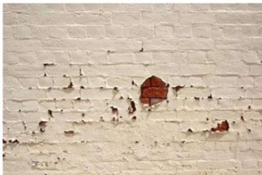
16: East facade showing 'rising damp'
