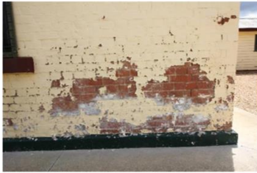
Evidence of rising damp at external wall
