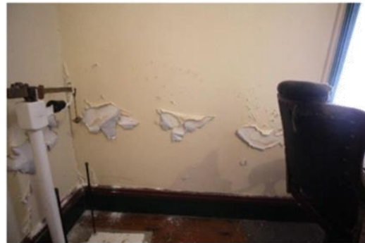
Evidence of rising damp at internal wall
