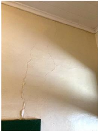
111: Hall - cracking at walls
