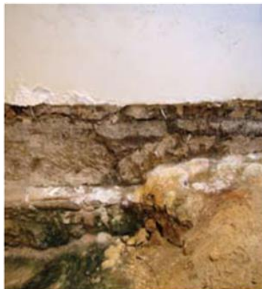
Figure 53 Damaged plaster on a damp wall; the dampness is indicated by green algae and white salts crystallising on the stonework and fill below. The recent plaster is decaying because it contains gypsum.
