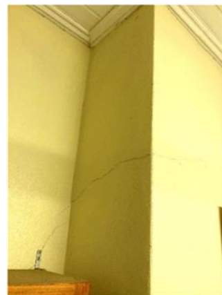
107: Entry Room – cracking at walls
