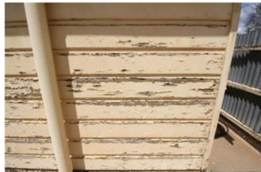
65: Deteriorated weatherboards
