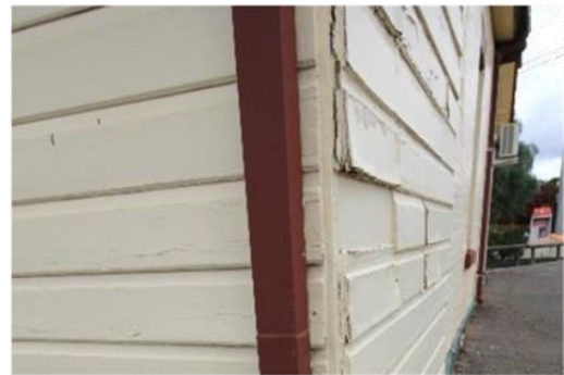
Evidence of deteriorated cladding at external wall
