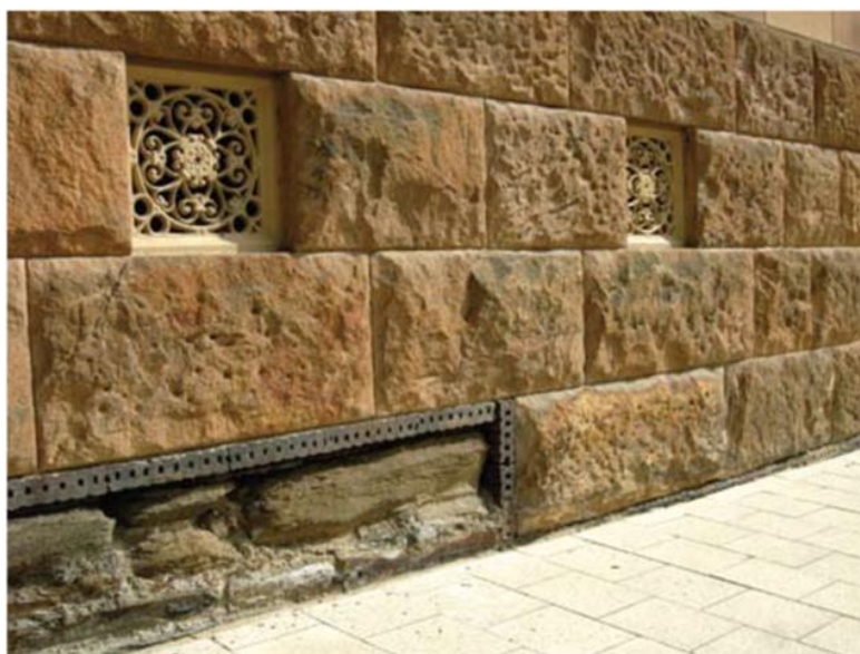
Figure 34 Stonework below the DPC needs attention as salts accumulate and the mortar and bluestone erode. In the first instance sacrificial treatments should be used to manage the problem. The 1879 ceramic DPC is doing an excellent job of protecting the sandstone above it, although where it steps down the slope it is compromised by hard paving that is laid too high, allowing splash onto the stone (see Box 2: Location of DPCs ).
