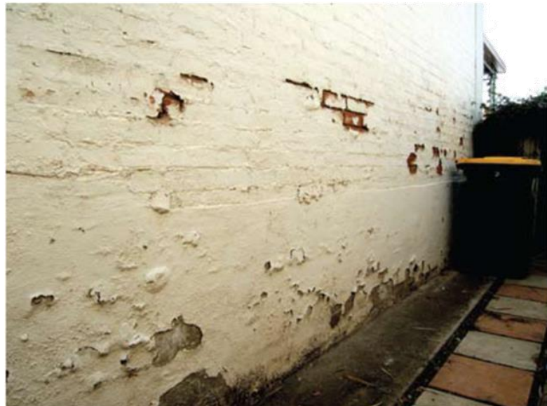
Figure 54 Failure of an acrylic paint coating due to salt damp. The bottom part of the wall is rendered in cement, which has contributed to the damp rising further due to its relative (but not total) impermeability. Decay of the brickwork is focussed where the paint film fails because that's where salt crystallises as moisture evaporates. The paint and the render should be removed and replaced with a more vapour-permeable coating such as limewash.
