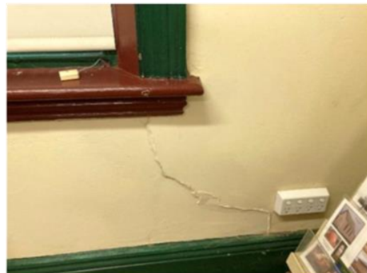
Evidence of movement cracking at internal wall
