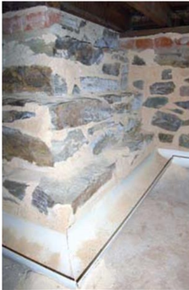
Figure 27 Semi-circular sections of PVC piping catch salt and other debris from sacrificial plasters and mortars on the walls beneath the floor of a church. Bedded on the same sacrificial mortar mix as that used for the walls, the pipes prevent the recirculation of the salts through the soils below and are cleaned out annually. White salts are visible on the stones in the centre of the photograph.
