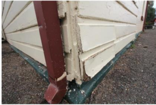
35: Deteriorated weatherboards north wall
