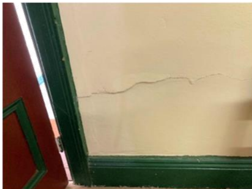
Evidence of movement cracking at internal wall
