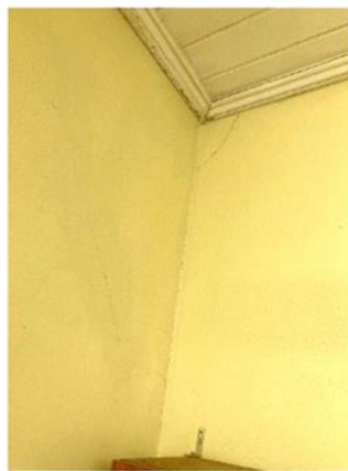
106: Entry Room – cracking at walls
