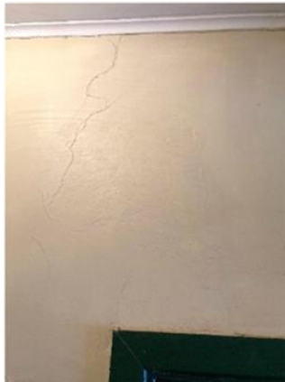
112: Hall - cracking at walls
