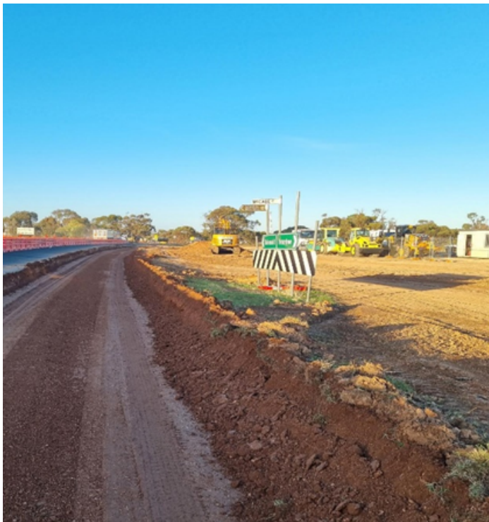
Upgrade of Ivanhoe Road / McCabe St Intersection shoulder preparation works April 2025
