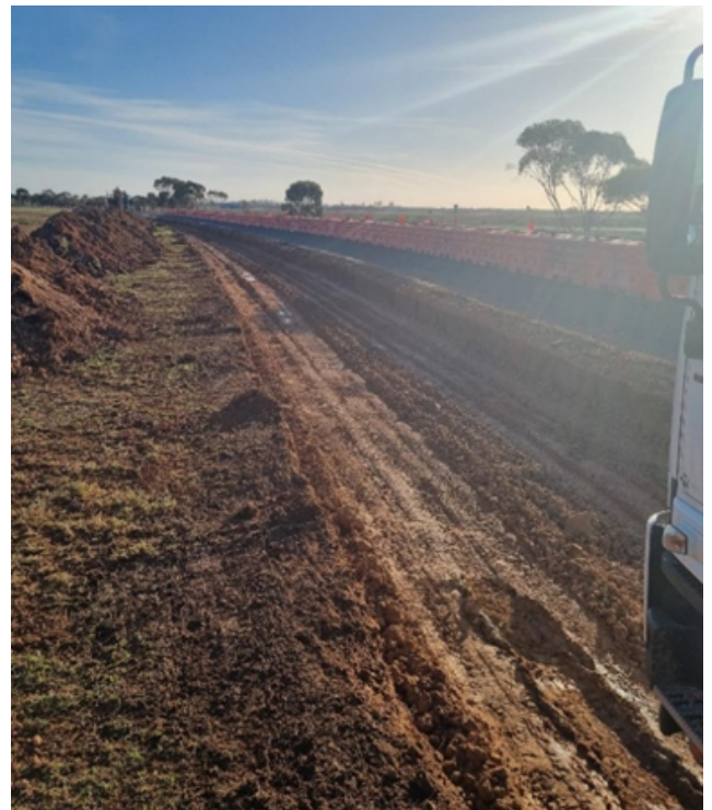
Upgrade of Ivanhoe Road / McCabe St Intersection shoulder preparation works April 2025
