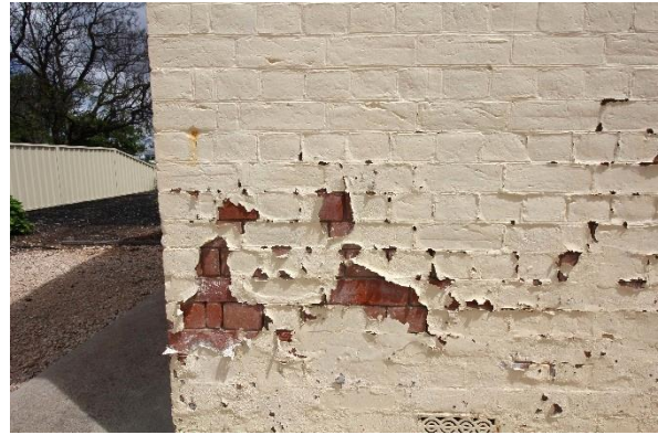
19: South facade showing 'rising damp'
