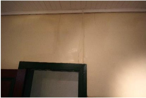
124: Robinvale Room - cracking at walls
