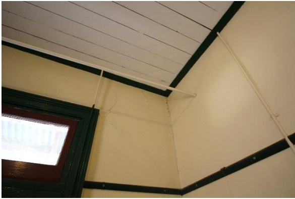
75: Nurses display structural tie rod / cracking
