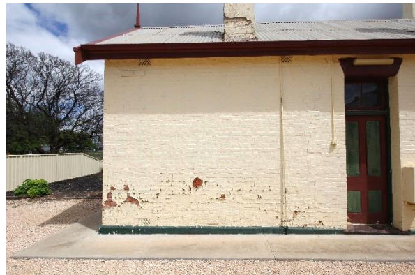
15: East facade showing 'rising damp'
