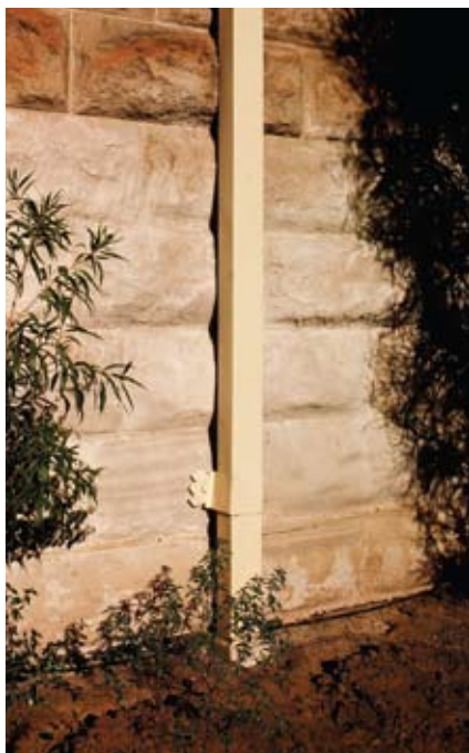
Figure 24 Garden beds against walls almost guarantee salt damp problems. Here the DPC was buried by 300 mm of soil — five courses of sandstone have been severely damaged.
