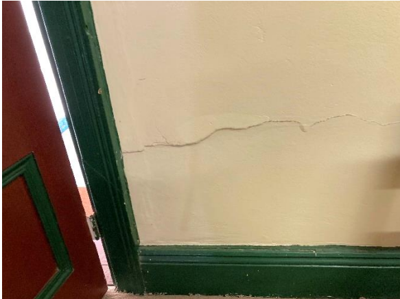
Evidence of movement cracking at internal wall
