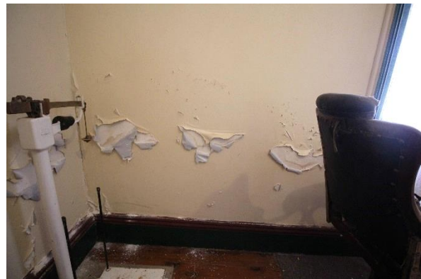
Evidence of rising damp at internal wall
