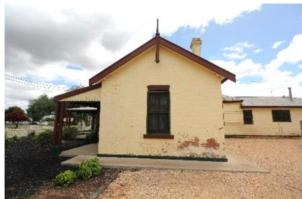
17: South facade showing 'rising damp'
