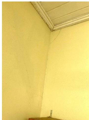
106: Entry Room – cracking at walls
