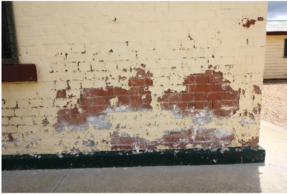
Evidence of rising damp at external wall
