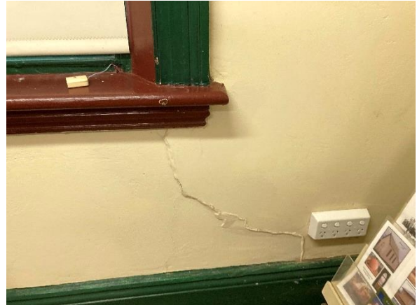
Evidence of movement cracking at internal wall
