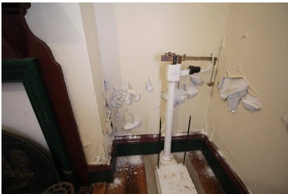
Evidence of rising damp at internal wall
