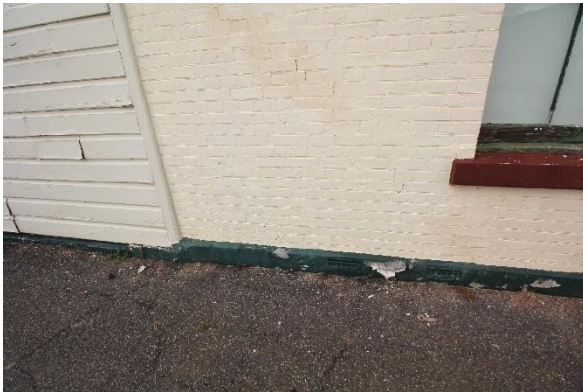
37: North facade - brickwork deteriorated at base
