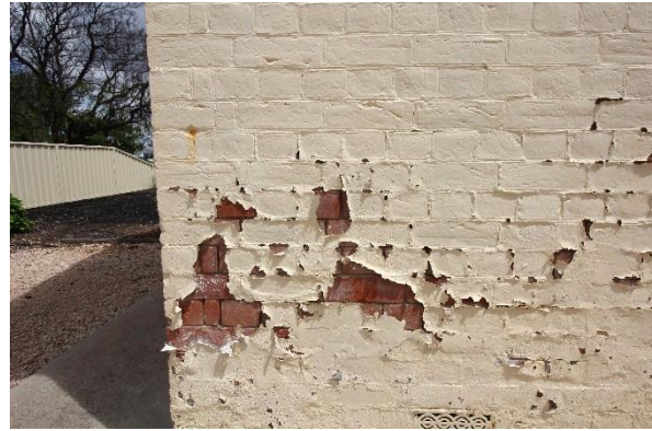
Evidence of rising damp at external wall
