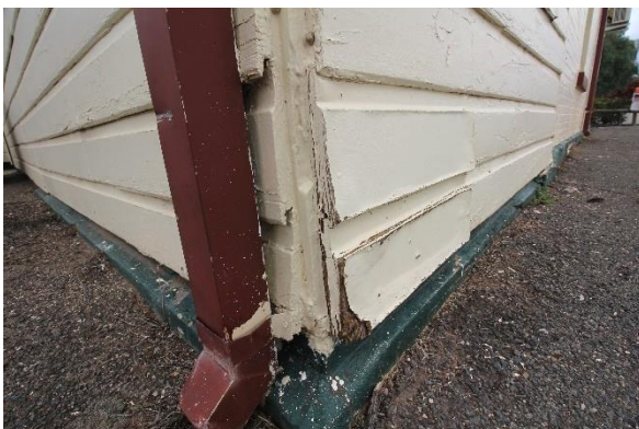
Evidence of deteriorated cladding at external wall
