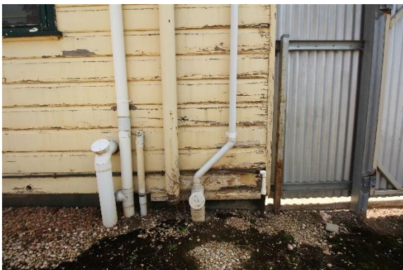
5: View of deteriorated weatherboards
