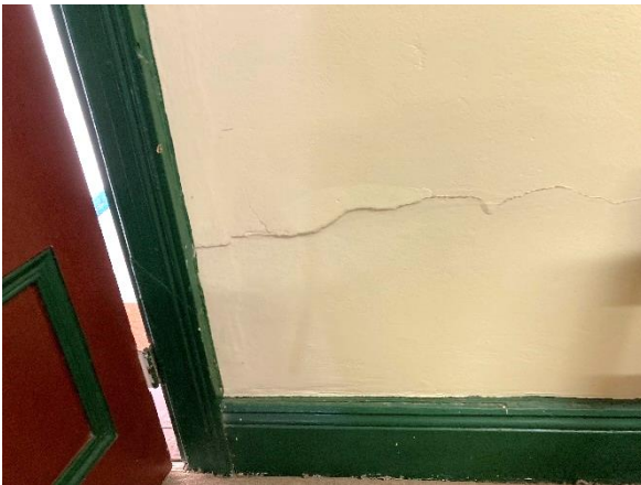
103: Entry Room – cracking at walls
