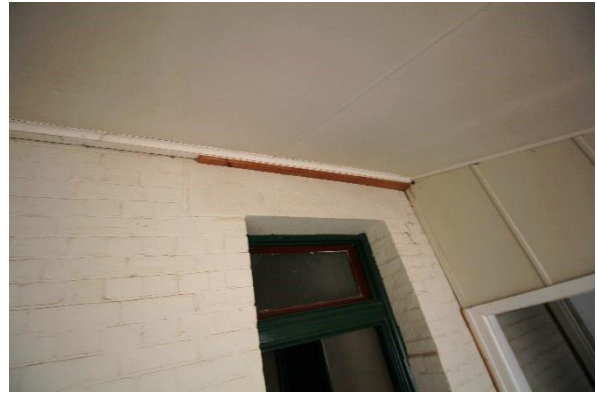
145: Infill verandah cracking at wall
