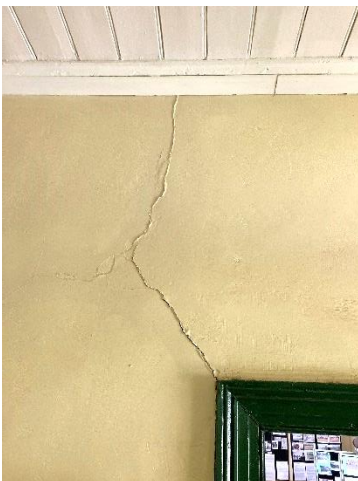
105: Entry Room – cracking at walls
