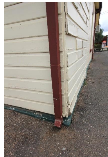
34: Deteriorated weatherboards north wall
