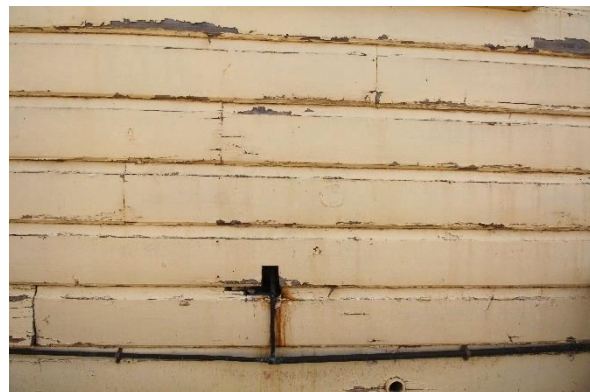
6: View of deteriorated weatherboards
