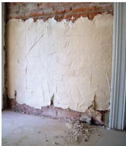
Figure 32 Absorbent poultice shortly after application to an interior wall from which plaster has been removed. The poultice is left on the wall until it is dry, which may take 2–3 weeks depending on weather conditions.
