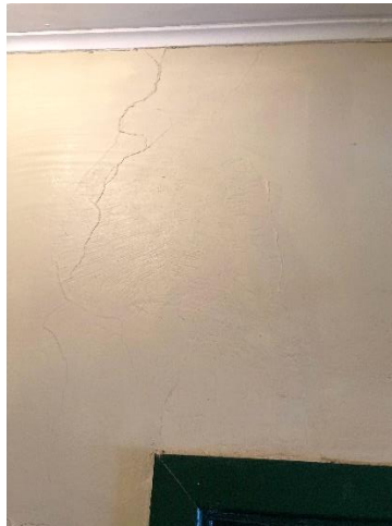
112: Hall - cracking at walls
