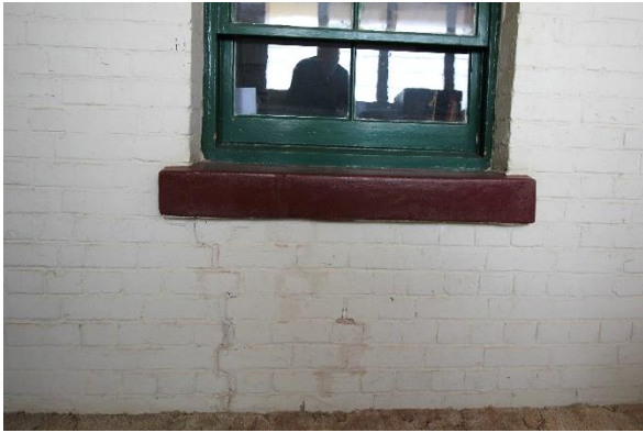
144: Infill verandah cracking at wall
