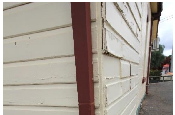
Evidence of deteriorated cladding at external wall
