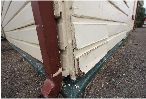
35: Deteriorated weatherboards north wall
