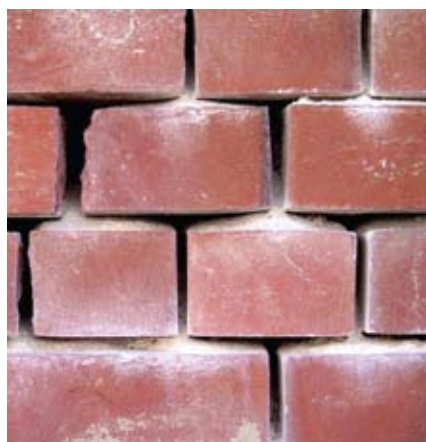
Figure 18 Extensive loss of lime mortar due to salt attack. The bricks remain sound — protected by the weaker mortar. Any further mortar loss risks local collapse of the brickwork. Successful repair may require dismantling and reconstruction as is done when undersetting (See Section 16.1).
