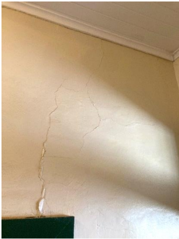
111: Hall - cracking at walls
