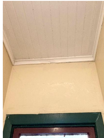
113: Hall - cracking at walls
