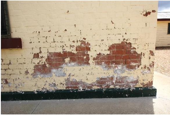
18: South facade showing 'rising damp'
