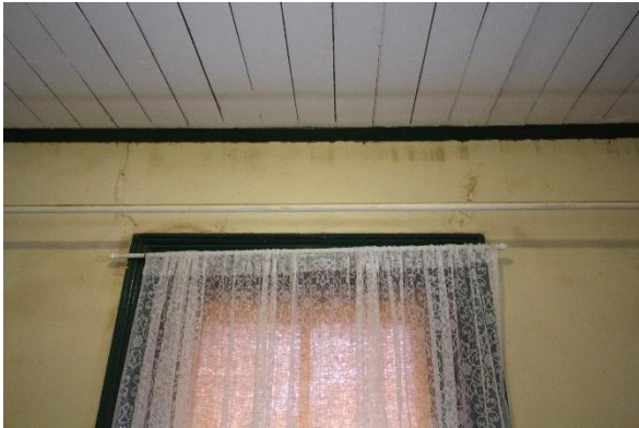
77: Nurses display structural tie rod / cracking
