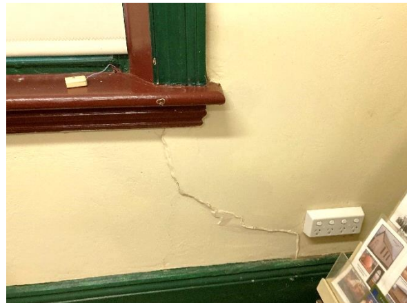
104: Entry Room – cracking at walls
