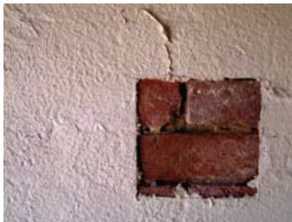
Figure 33 A square section of dried poultice has been cut out for chemical analysis. Sampling of the same point during subsequent cycles of poulticing is aided by a marker such as the galvanised nail in the bottom left of the 'window'.
