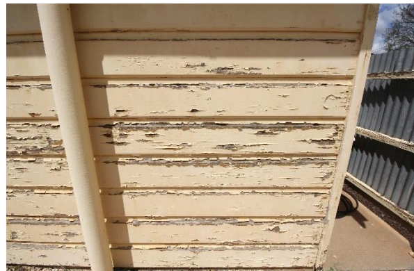
65: Deteriorated weatherboards
