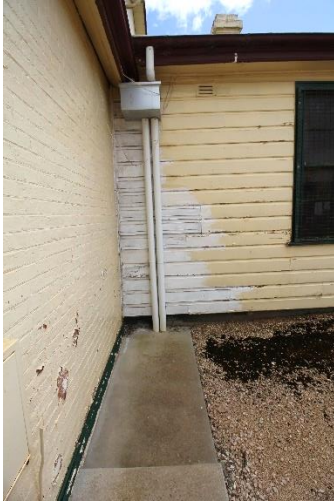
11: View of junction – b/w original + extension
