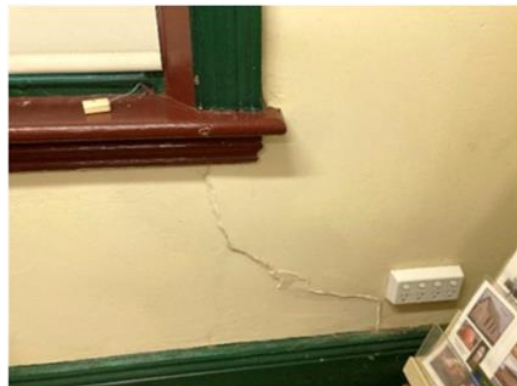
Evidence of movement cracking at internal wall
