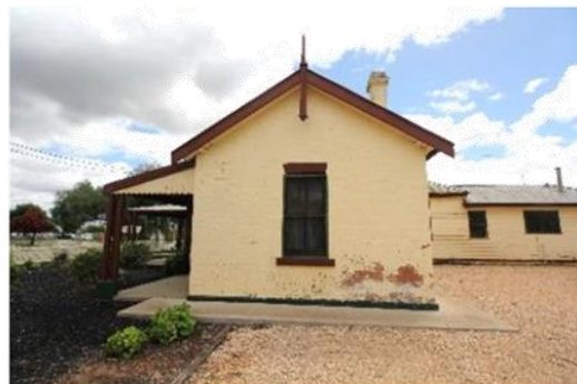
17: South facade showing 'rising damp'
