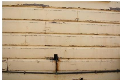
6: View of deteriorated weatherboards
