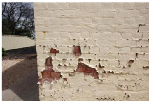
19: South facade showing 'rising damp'
