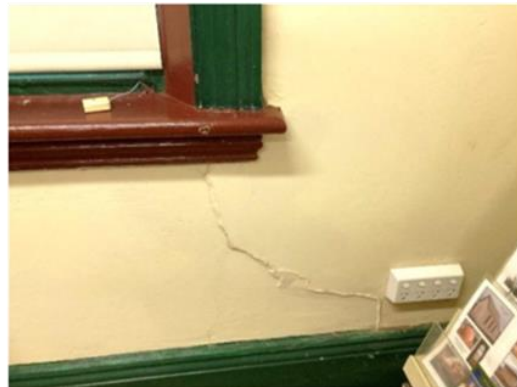
104: Entry Room – cracking at walls
