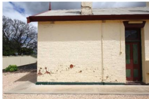
15: East facade showing 'rising damp'
