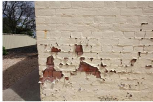
Evidence of rising damp at external wall
