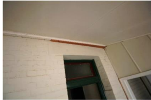
145: Infill verandah cracking at wall
