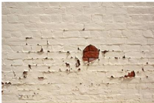
16: East facade showing 'rising damp'
