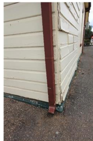
34: Deteriorated weatherboards north wall
