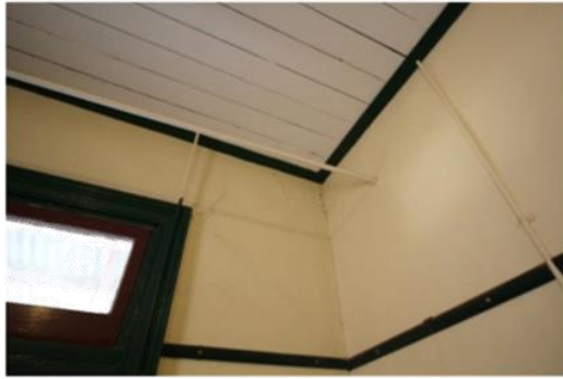
75: Nurses display structural tie rod / cracking
