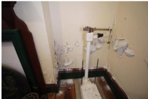
Evidence of rising damp at internal wall
