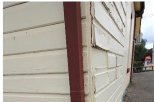
Evidence of deteriorated cladding at external wall
