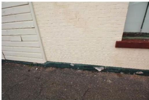
37: North facade - brickwork deteriorated at base
