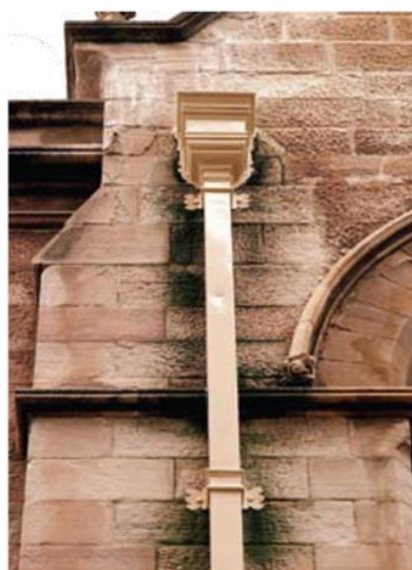
Figure 14 (right) Two examples of falling damp. Overflow from the blocked rainwater head is made apparent by dark green algae. The coping above the rainwater head is allowing water through to the stones below. Salt attack is causing these stones, above and to the left of the rainwater head, to decay.
