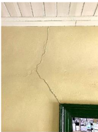
105: Entry Room – cracking at walls
