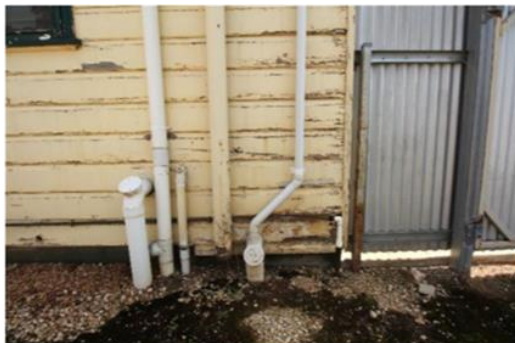
5: View of deteriorated weatherboards
