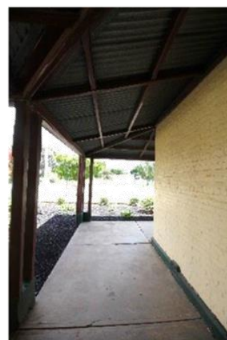
50: Concrete paving at verandah
