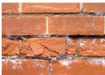
Figure 5 Salt attack in bricks causing disruption and loss of the fireskin, the harder outer surface that develops during firing in the brick kiln.
