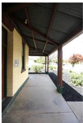
48: Concrete paving at verandah
