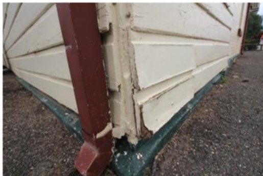
Evidence of deteriorated cladding at external wall
