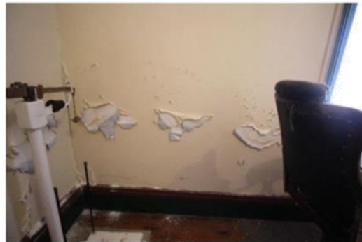
Evidence of rising damp at internal wall
