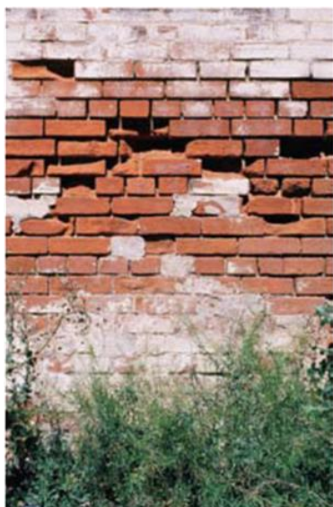
Figure 2 Typical salt damp damage in Adelaide, with decay of the bricks extending from about 0.5 to 1.2 metres above ground. There are no obvious signs of salt because it has been washed off by rain. Paler (underfired) bricks are more susceptible to salt attack than the darker, more well-fired ones.
