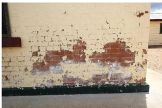
18: South facade showing 'rising damp'
