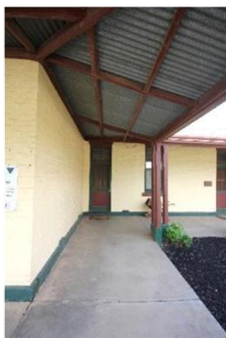
49: Concrete paving at verandah
