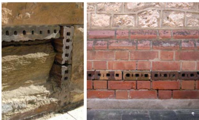
Figures 9 and 10 Hard burnt and glazed ventilating ceramic tiles and bricks. Made for the purpose, these are among the best dampcourses ever used, particularly the example at left from 1879. At right is a 1930s example which (together with its adjacent brickwork) is a remedial undersetting of an 1840s church of rubble limestone. Both examples were laid with open perpendicular joints to prevent damp travelling through the permeable mortar. In both cases salt attack is damaging the masonry below the DPCs — and each building will need treatments to control the salts (see Sections 13 & 14).
