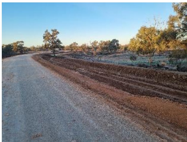
Pictures McCabe Street Road widening construction works July 2025
