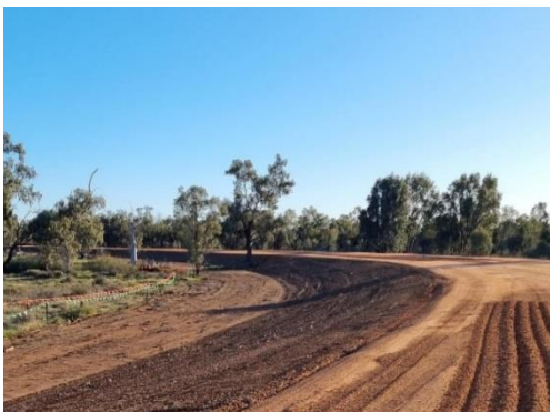
August 2025 McCabe Street facing Southeast
