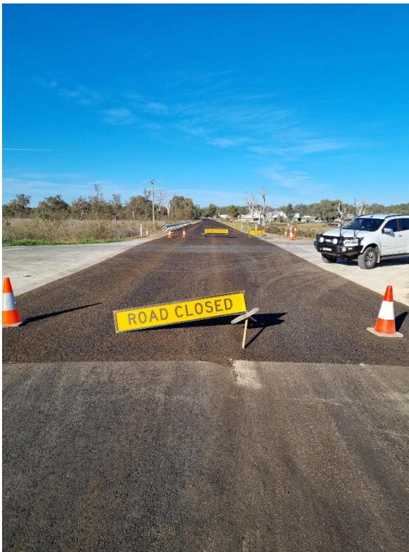
September 2025 new asphalt to 2 coat spray seal driving surface finish McCabe Street
