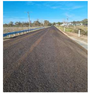
New asphalt to 2 coat spray seal driving surface finish McCabe St
