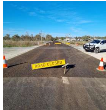
New asphalt to 2 coat spray seal driving surface finish McCabe St
