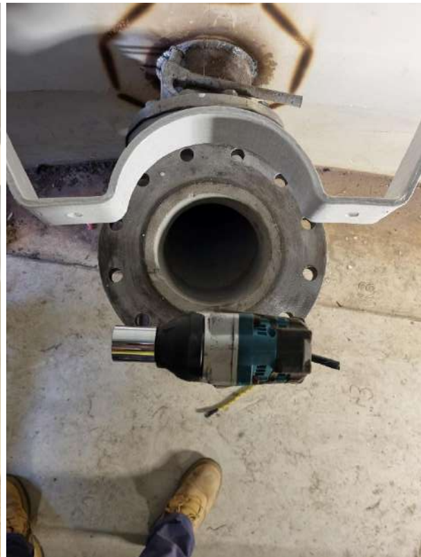
Photo of new internal rising main elbow flange bracket November 2025
