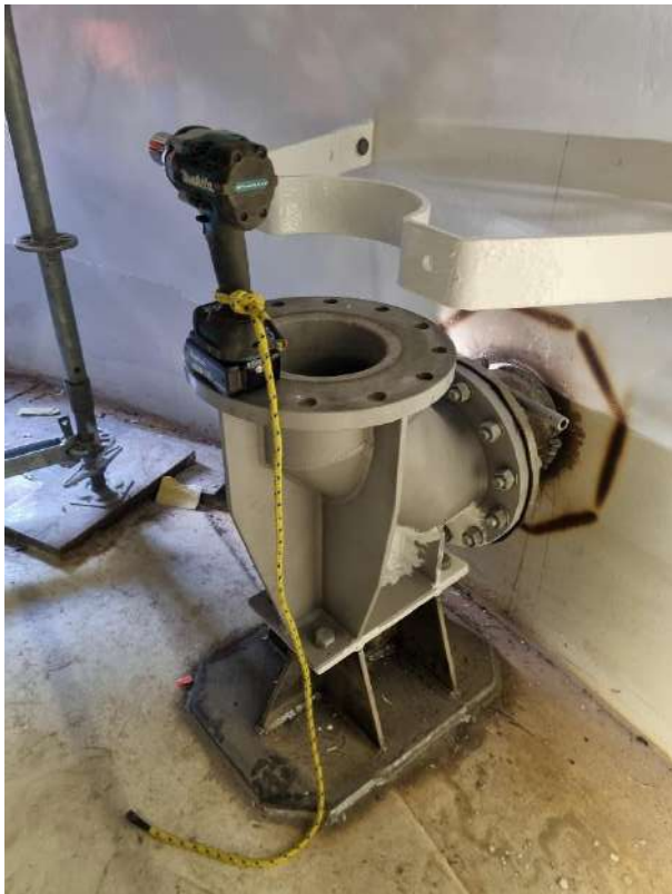
Photo of new internal rising main elbow flange November
