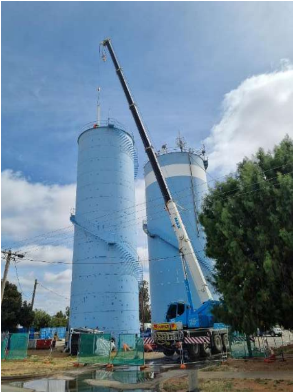
Photo of crane lowering replacement overflow pipe November Photo of replacement overflow pipe elbow November 2025
