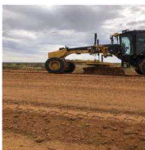
Figure 10 Oxley road maintenance grading
