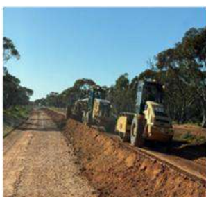
Figure 13 Tapalin mail rd maintenance grading
