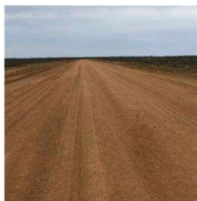
Figure 10 Oxley road maintenance grading
