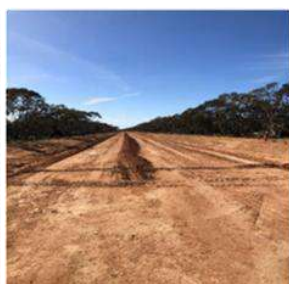
Figure 13 Tapalin mail rd maintenance grading
